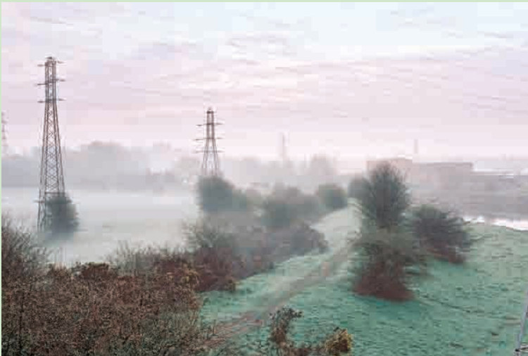
Infrastructure can impact on visual amenity of the land.
